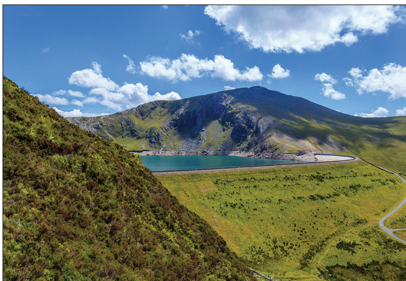
Figure 9b: Dinorwig hydroelectric power scheme, North Wales
