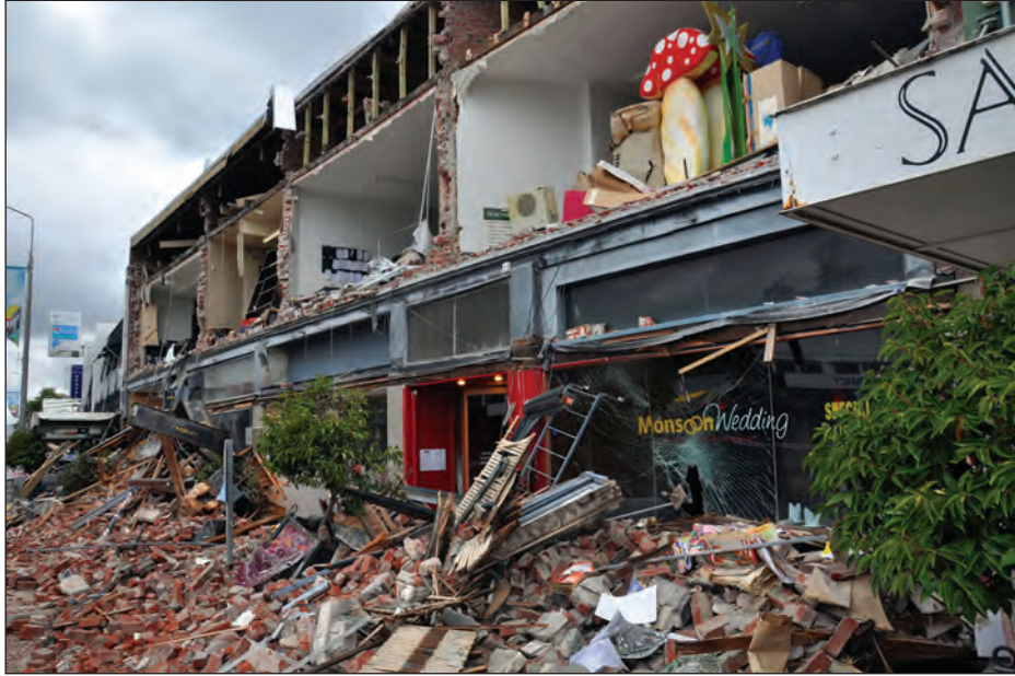
Photo 3.3 – Damage to homes and businesses in Christchurch after the 2011 earthquake
