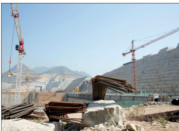
The construction site of the dam
